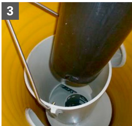
3 Insert the operating pipe in the base shaft with bayonet nut connector.
