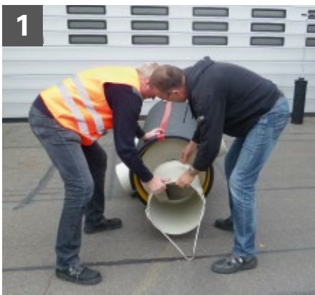
1 Inserting the sediment collector in the base shaft
