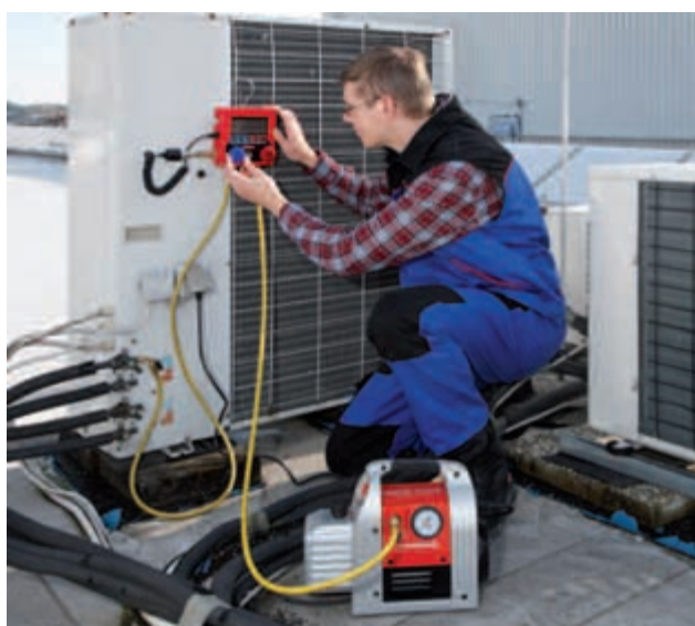
ROAIRVAC - vacuum pump in use with the digital manifold
