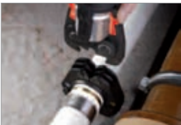
Gripping the pressing collar with intermediate jaws
