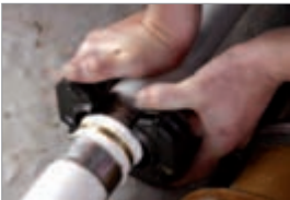
Gripping the pressing collar with intermediate jaws
