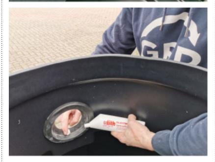
Step 9. Lubricate the rubbers of the inlet and outlet with the supplied lubricant.
